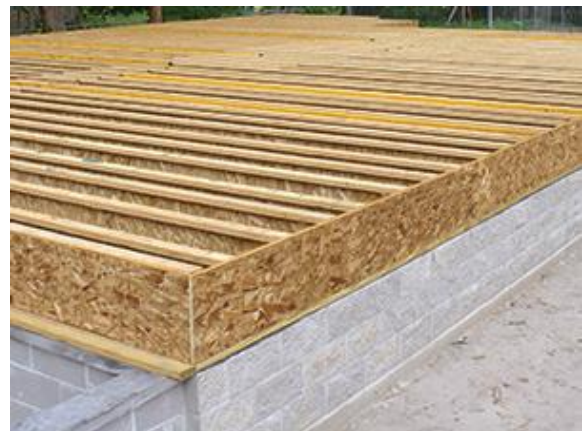
Figure 12: Stem Wall Foundation
