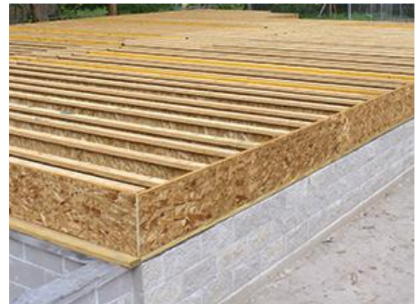
Figure 12: Stem Wall Foundation
