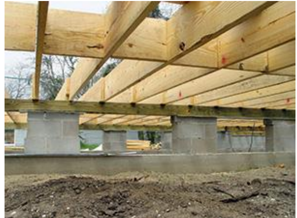
Figure 11: Pier and Beam Foundation
